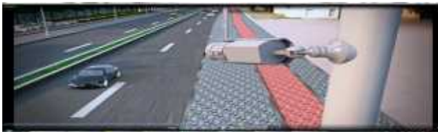
Traffic Monitoring Cameras
